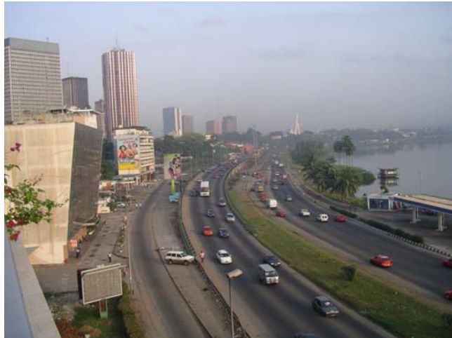
Boulevard General de Gaulle runs along the Lagoon
